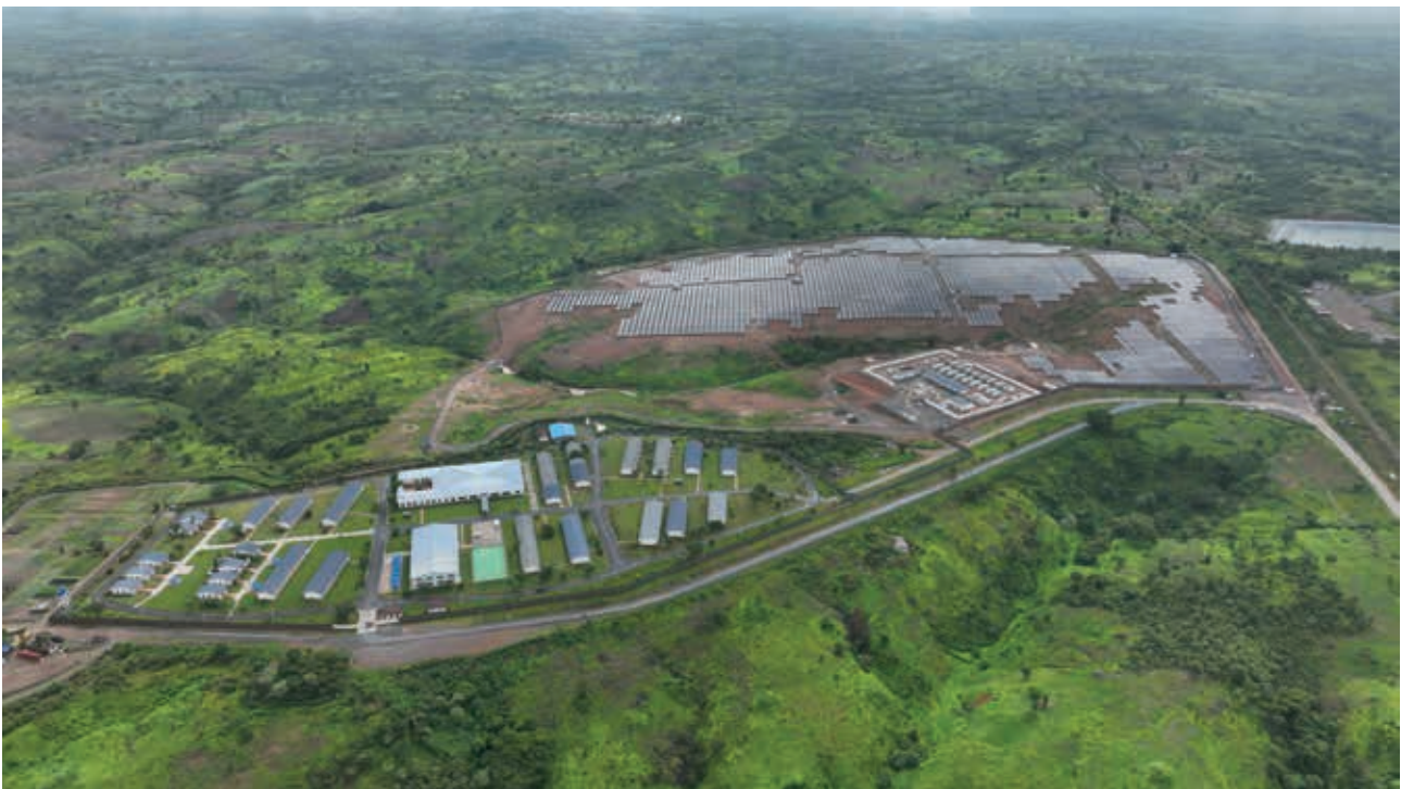
Photovoltaic-storage power stations at Kambove Mining
