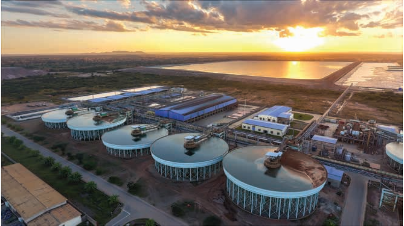
Leaching workshop of Luanshya Muliashi Leaching Plant
