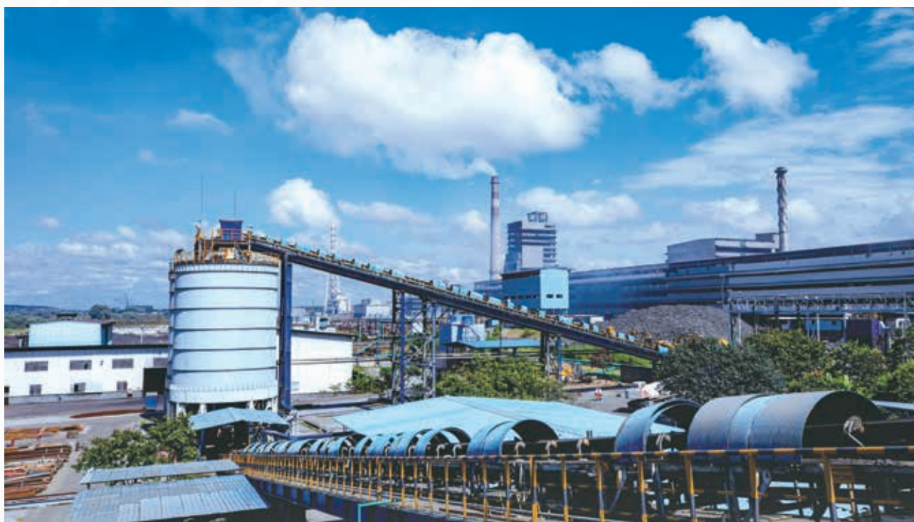
Part of CCS plant site
